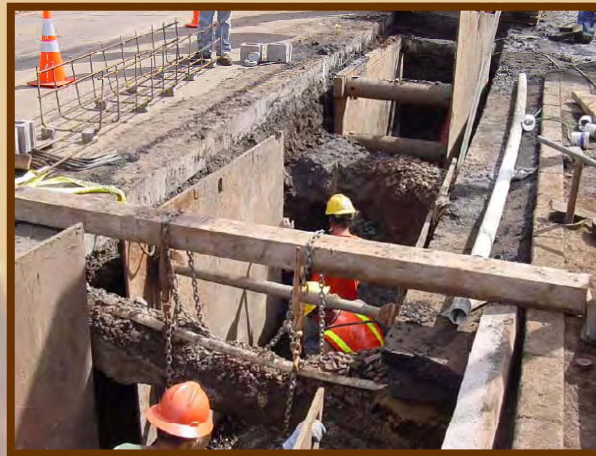
UTILITY CONFLICTS - The new sewerline crosses many existing utility lines, requiring field adjustments and concrete encasements.
