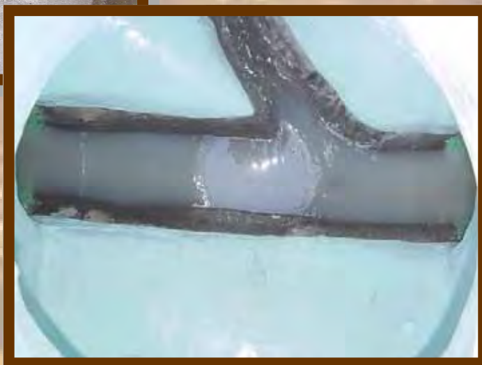
MANHOLE REHABILITATION - Existing sewer manholes were re-channelized (top left) and protected with an epoxy coating (bottom right).
