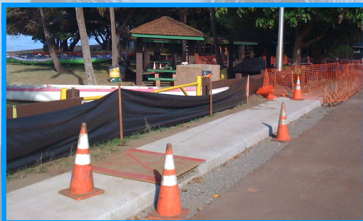
Photo left: silt fence prevents sediment and runoff from flowing to the ocean at Hanakao'o Beach Park.
