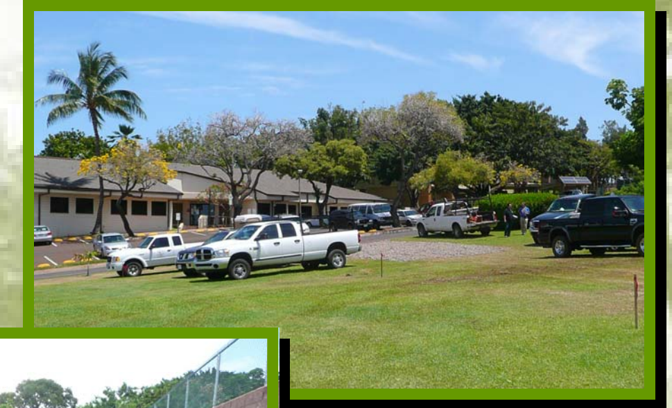
Photo Above - Entrance before construction. A temporary gravel apron was installed as an erosion control measure to prevent the tracking of sediment outside the construction area. Photo Left - New paved entrance and 25-stall parking lot.
