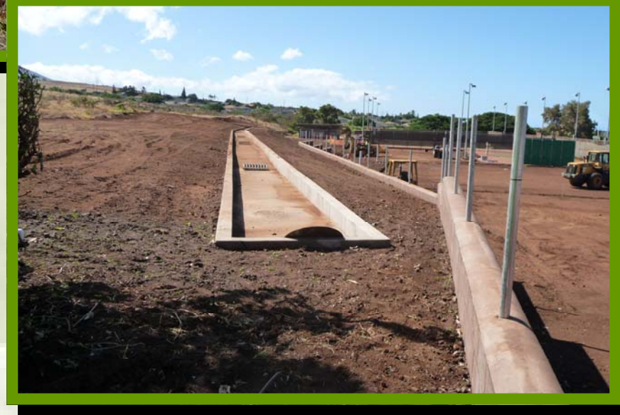
Photo Top - Undeveloped land owned by the State Department of Hawaiian Home Lands. Photo Bottom Right - New concrete drainage channel designed to capture off-site storm runoff. Photo Bottom Left - Special clog-resistant grated drain inlet.
