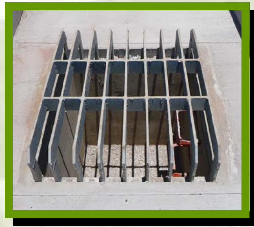
Photo Top - Undeveloped land owned by the State Department of Hawaiian Home Lands. Photo Bottom Right - New concrete drainage channel designed to capture off-site storm runoff. Photo Bottom Left - Special clog-resistant grated drain inlet.
