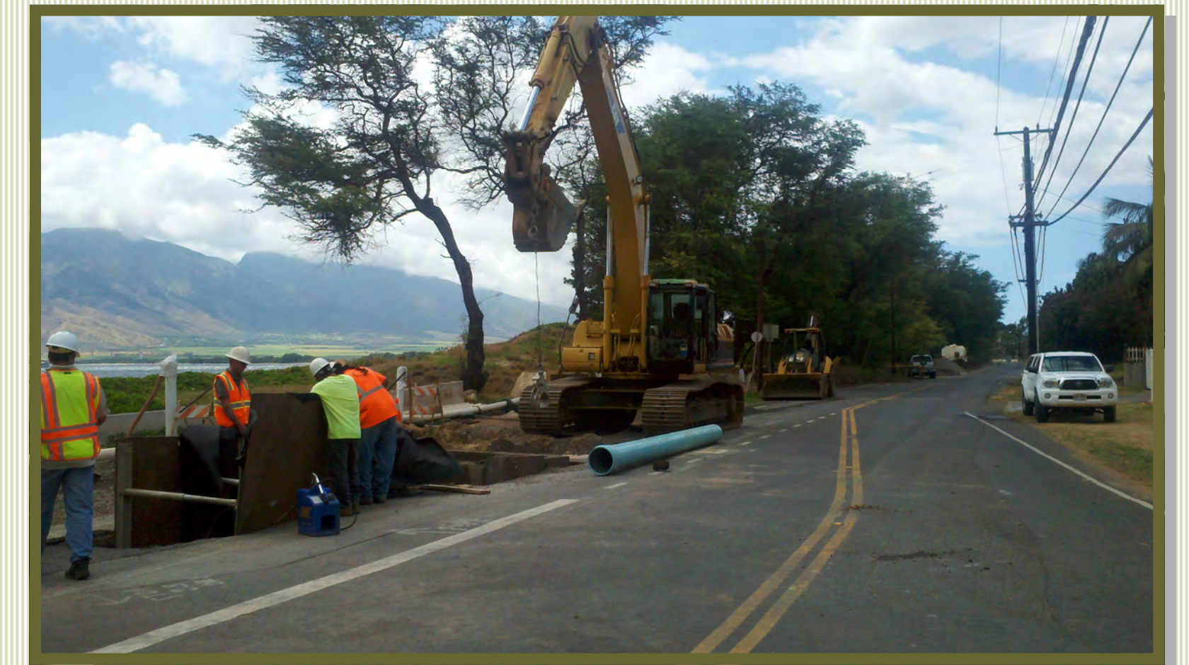
INSTALLING SEWERLINE - Force main being installed in South Kihei Road.
