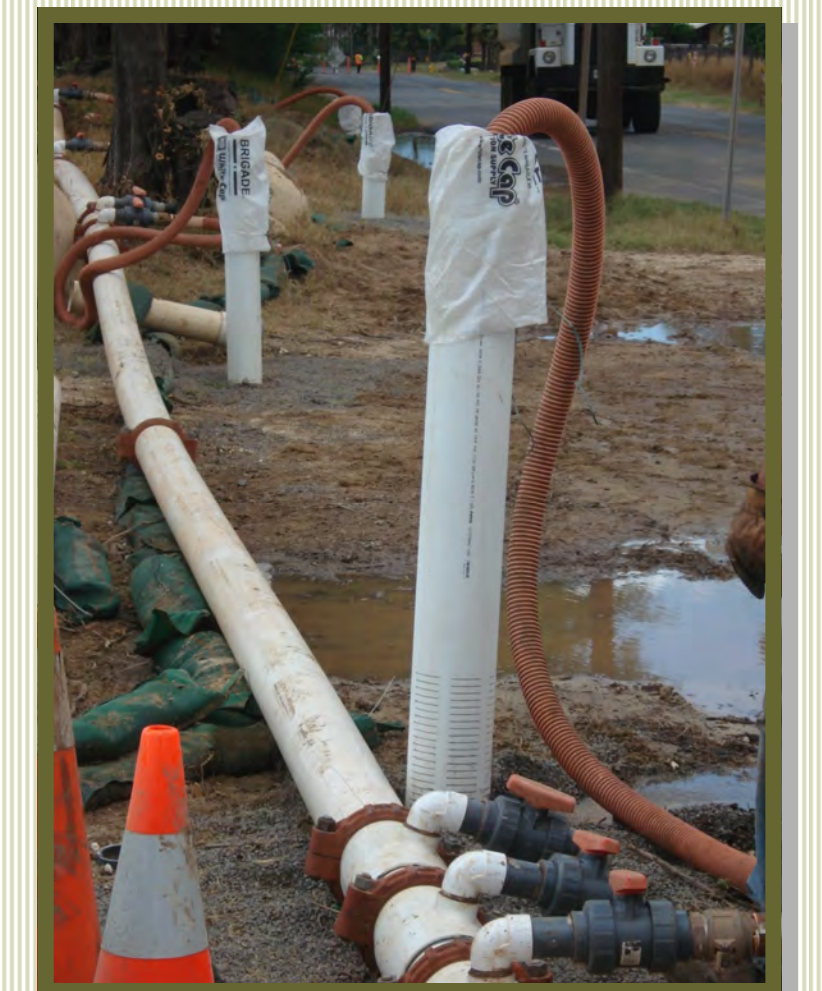
DEWATERING WELLS – A series of wells were used to temporarily lower groundwater.
