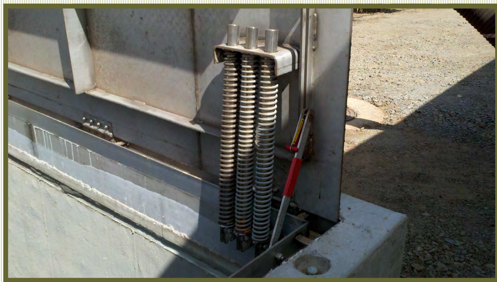
VAULT LID – Due to the 1,500-lb. weight of the lid, spring-loaded hinges were added for ease of opening.
