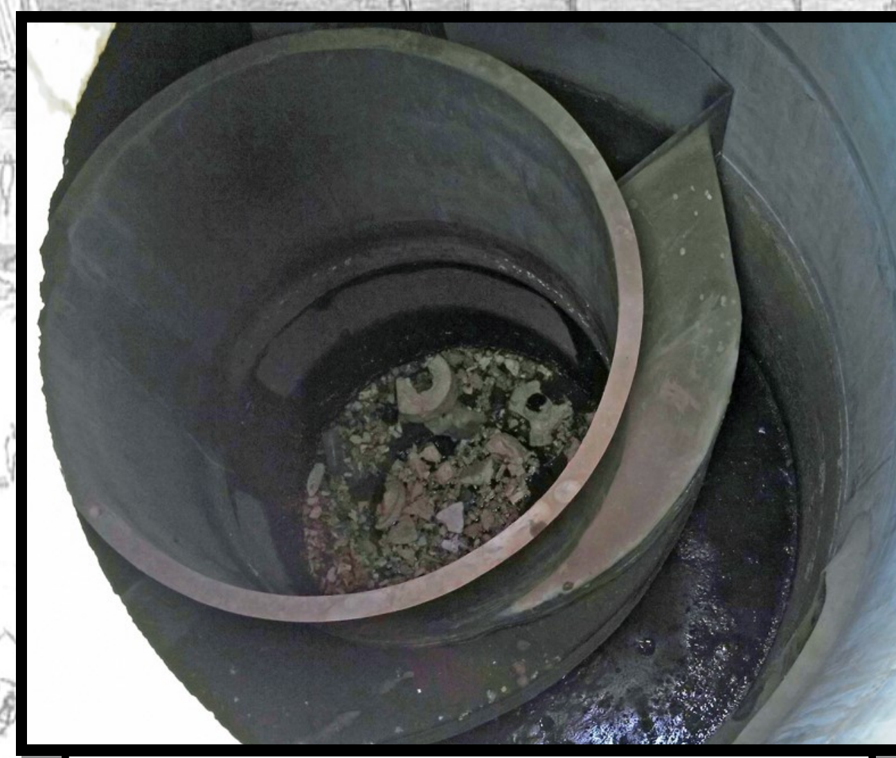
Debris Caught During Construction in Stormwater Filter
