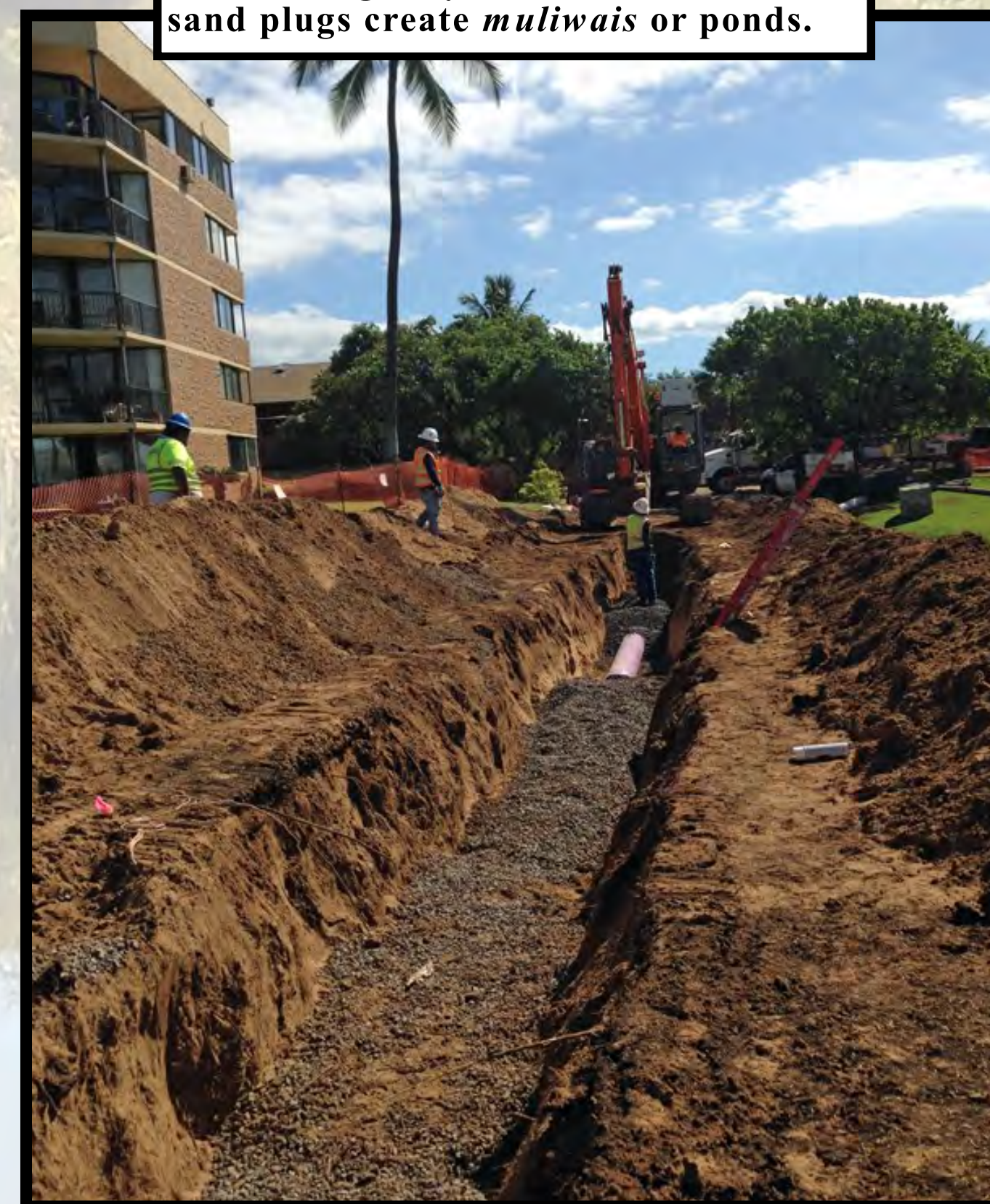
Waterline installation fronting the condominium properties.
