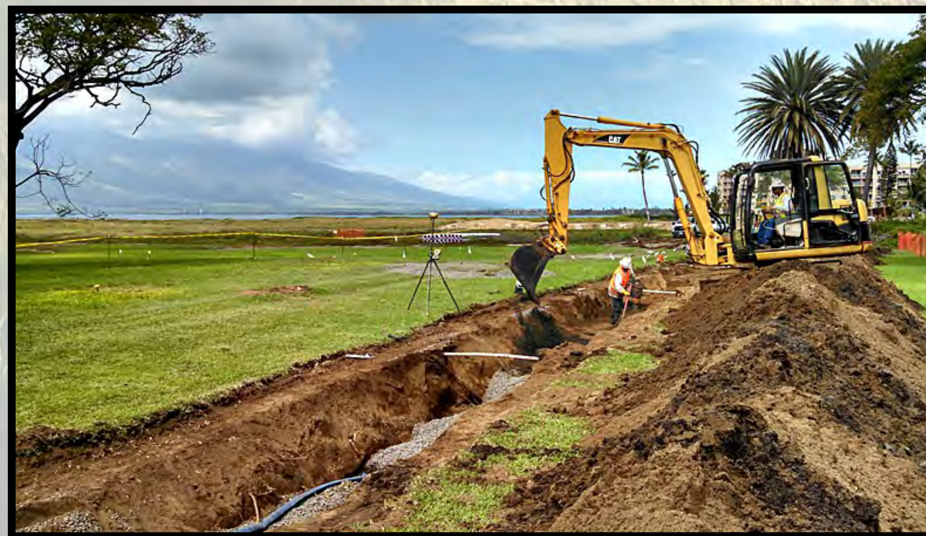
Backfilling trenches after installation of waterline at Waipuilani Park.
