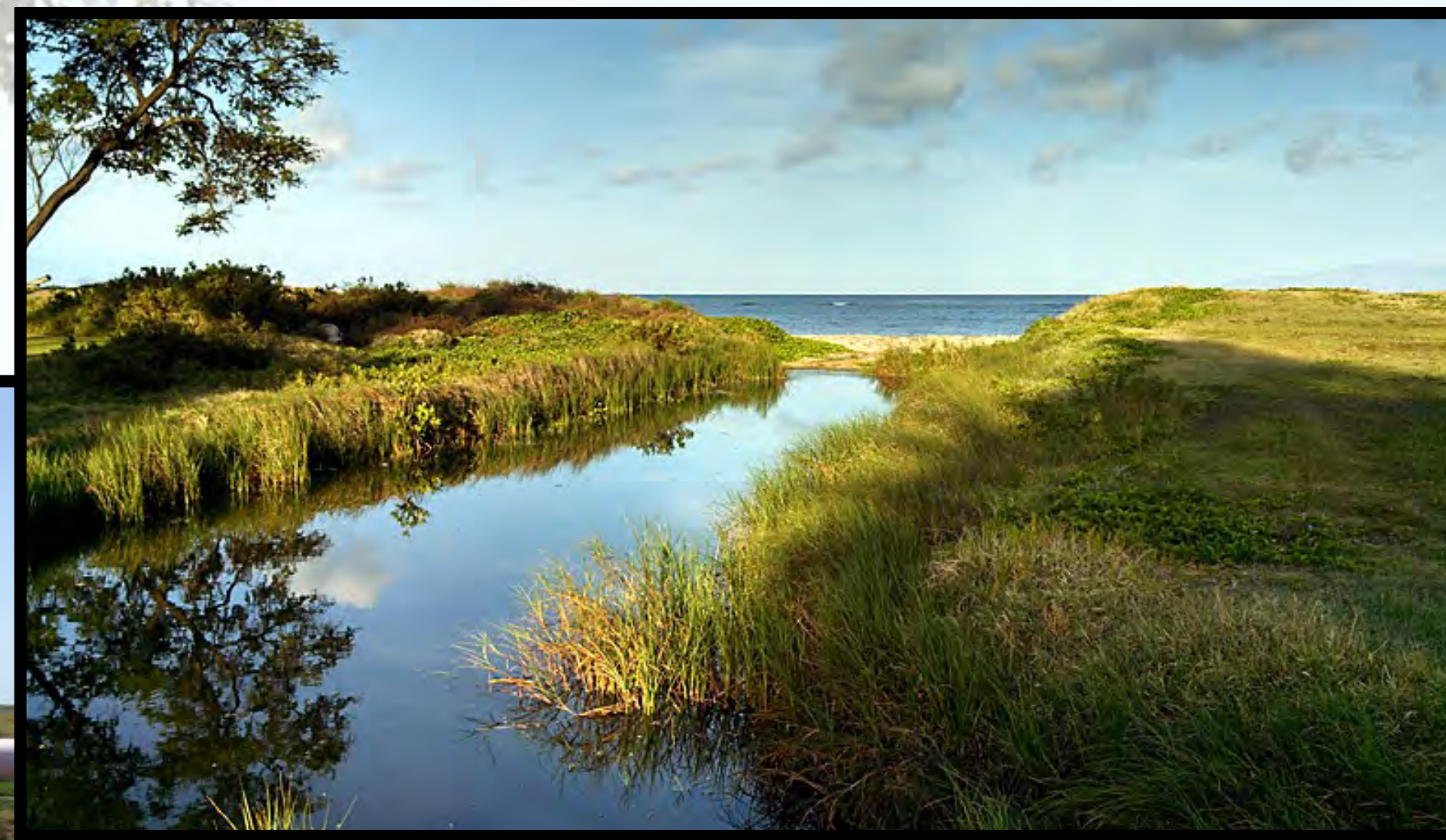
The waterline was installed using horizontal directional drilling under two drainageways where the shoreline sand plugs create muliwais or ponds.
