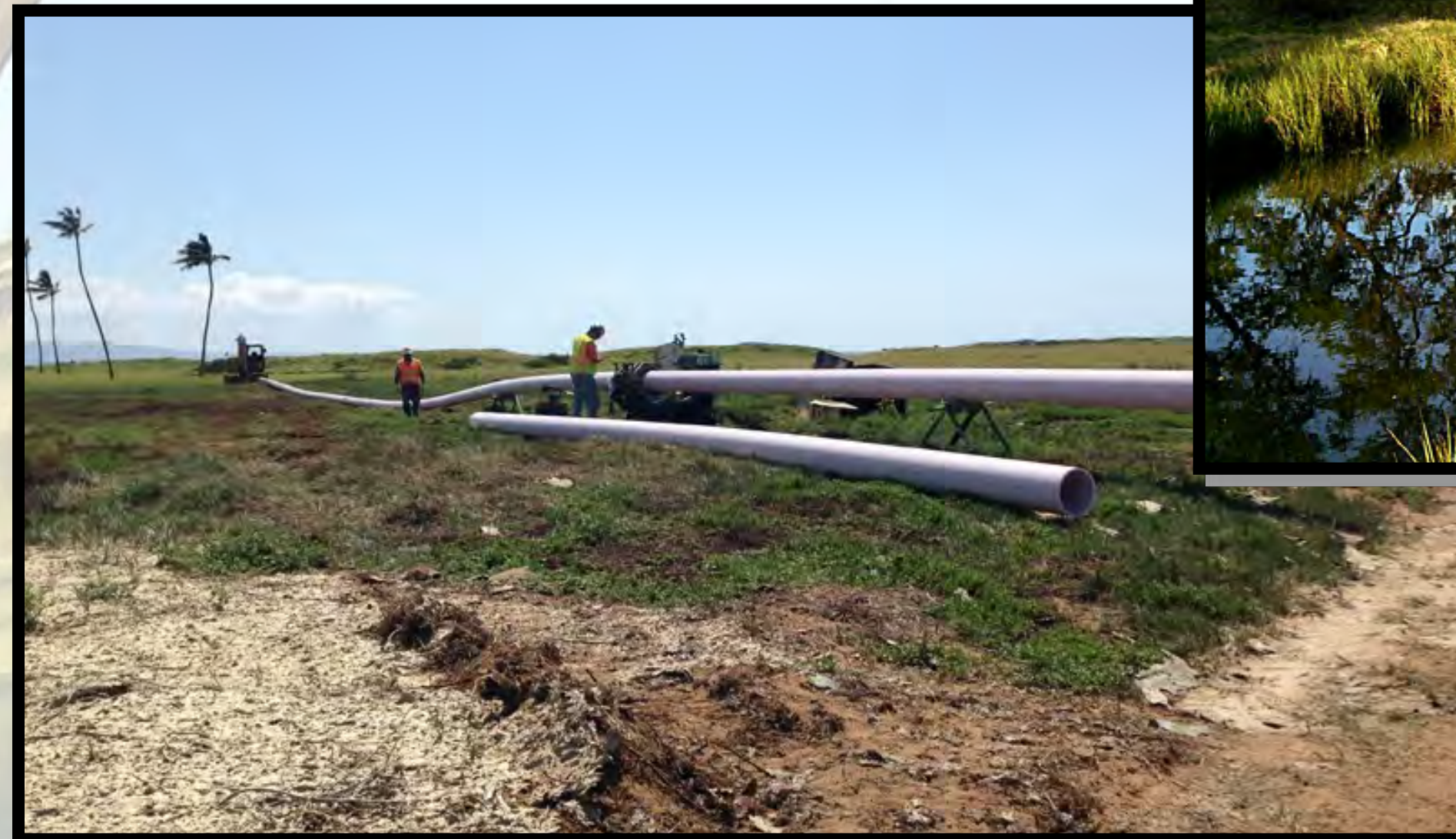
Fusing together lengths of PVC waterlines.
