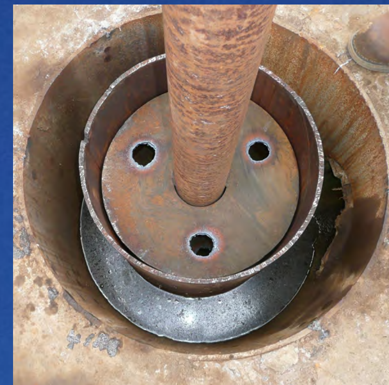
Mandrel in casing for alignment test.
