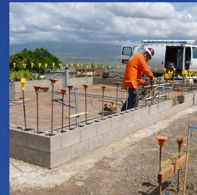
Setting starter courses of CMU block for building.
