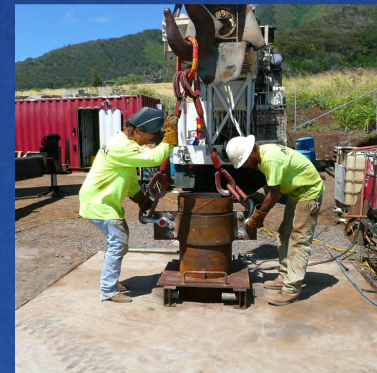
Removing lifting shackles during casing installation.
