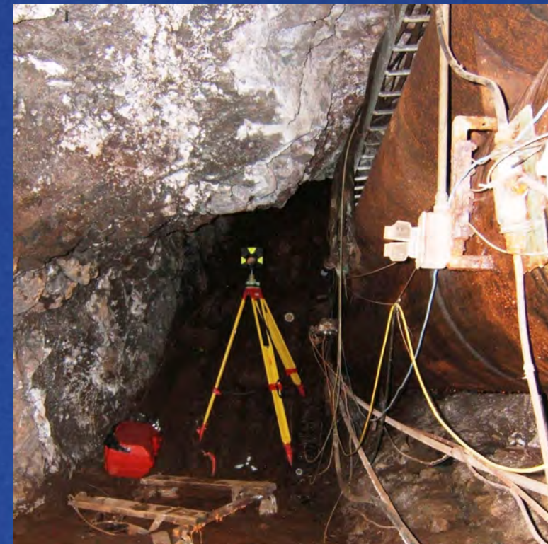
Setting survey control point in tunnel of Shaft 33.
