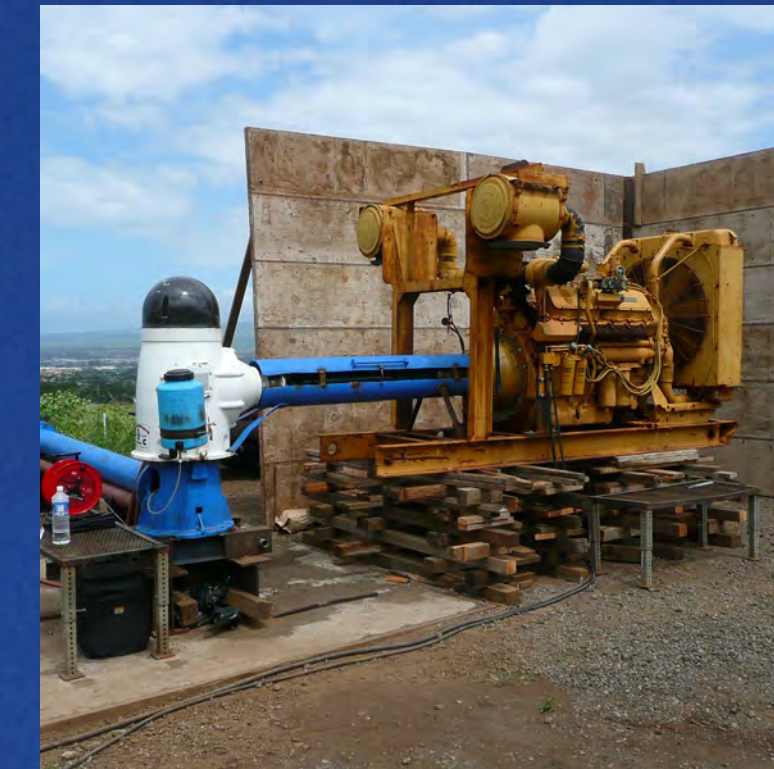
Right angle drive for pump powered by diesel engine.
