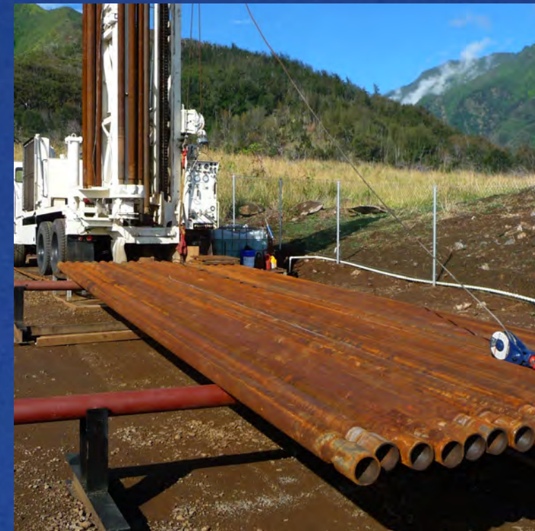
Drill pipe with drill rig.
