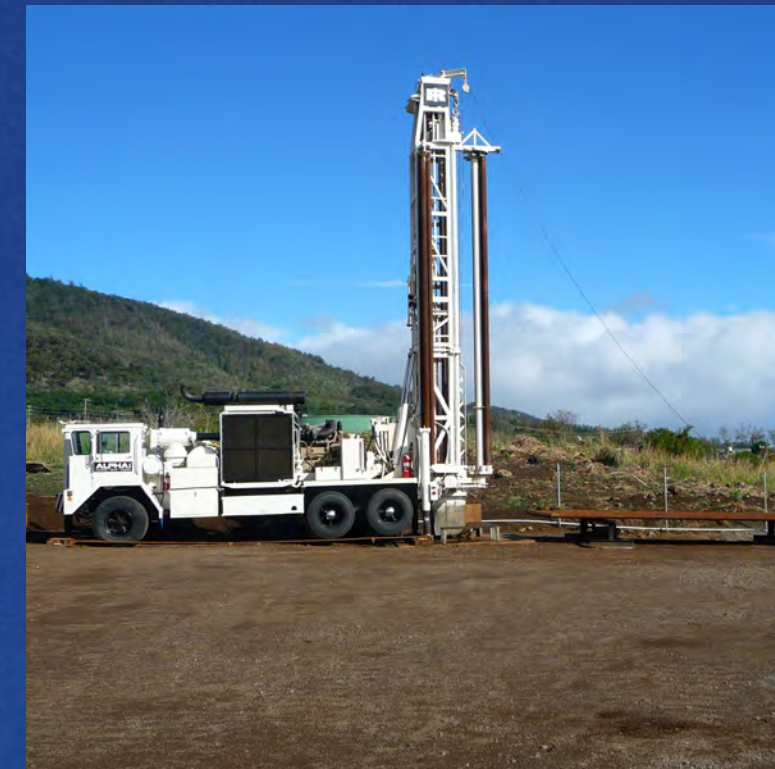
Rotary drill rig.
