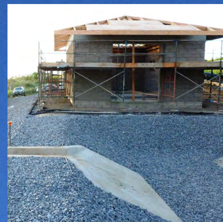
Drainage sump and building under construction.
