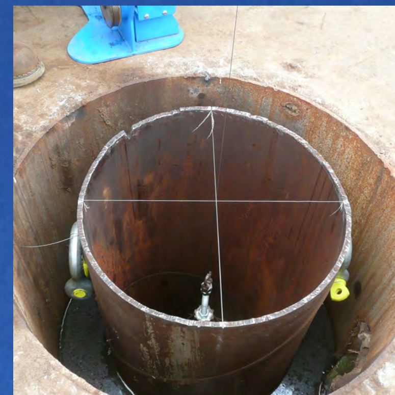
Measuring drift of plumb line for alignment test.
