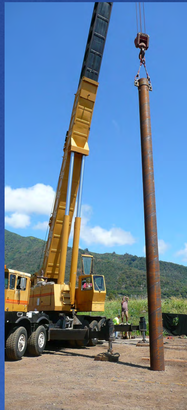
Installing 18-inch diameter steel casing.
