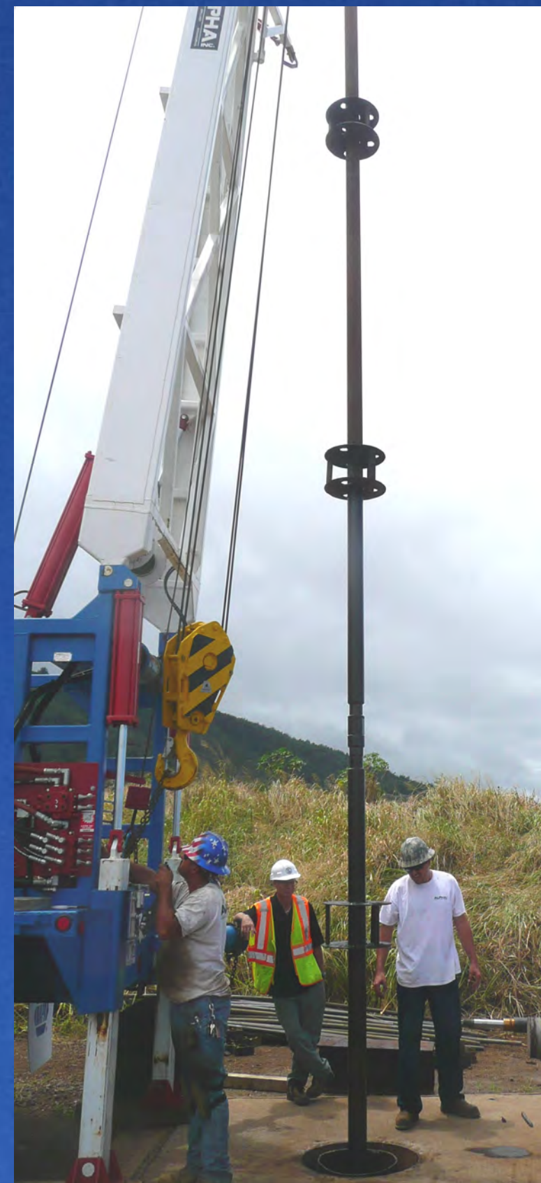
Lowering mandrel into casing for alignment test.
