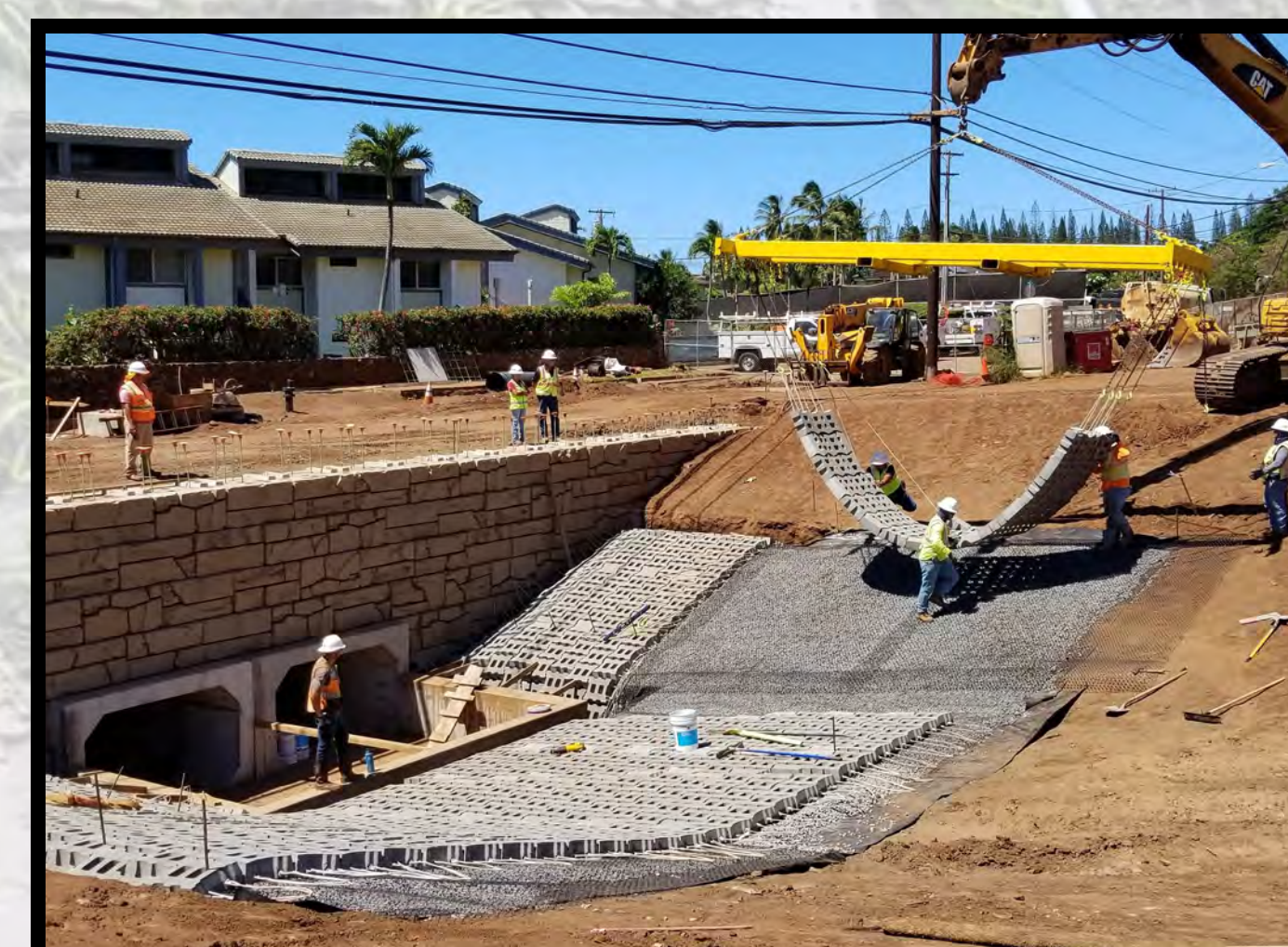
DURING: Installing articulated-block mats in the drainageway.
