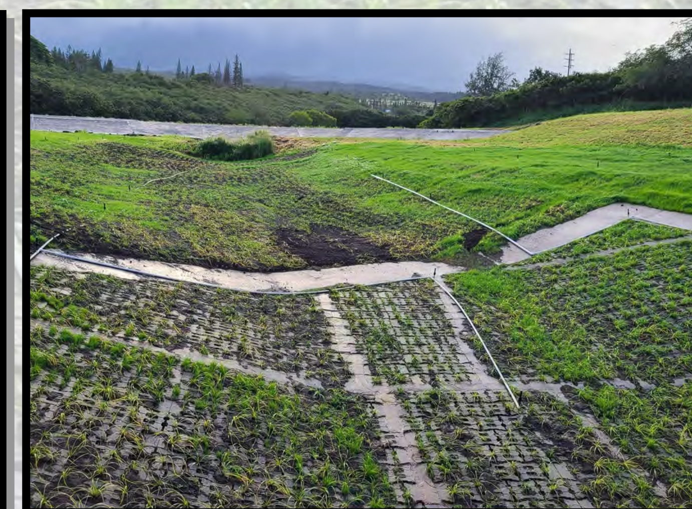
AFTER: Native grass planted in the stream & drainageway.
