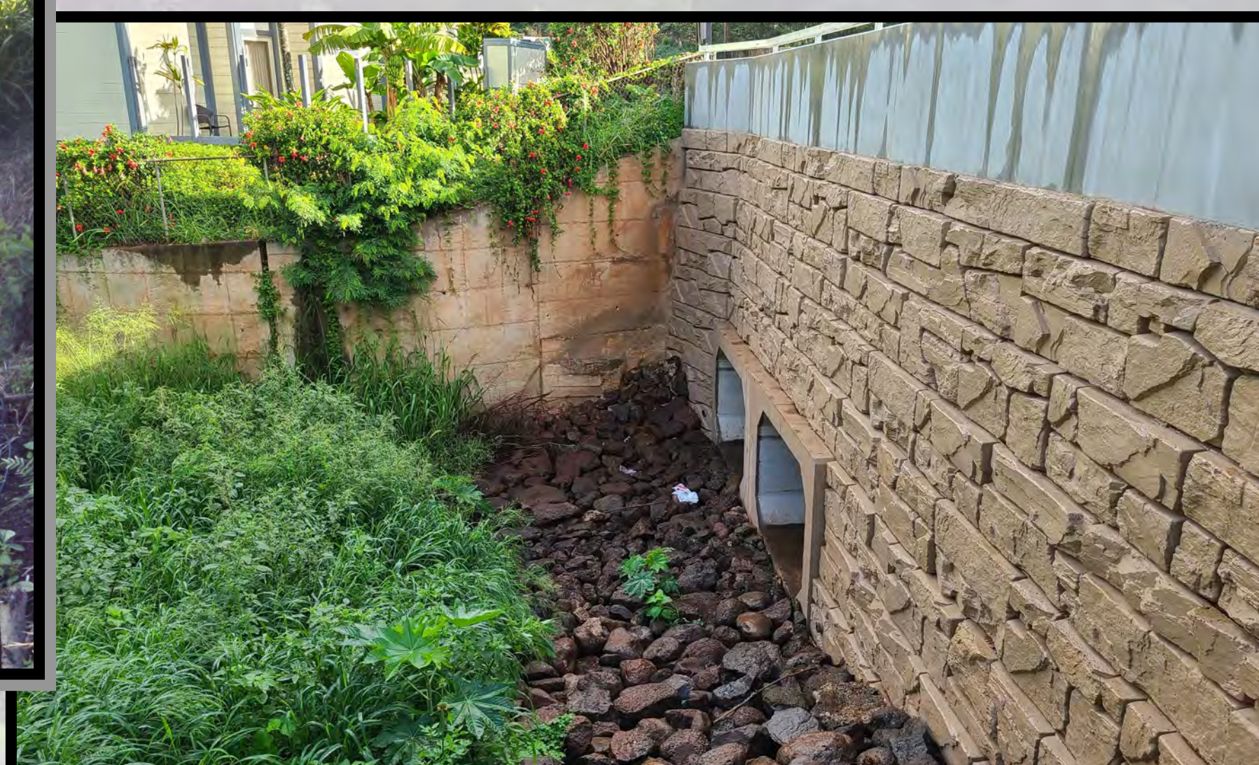
AFTER: New drainage way, featuring lowered precast drainage box culverts.
