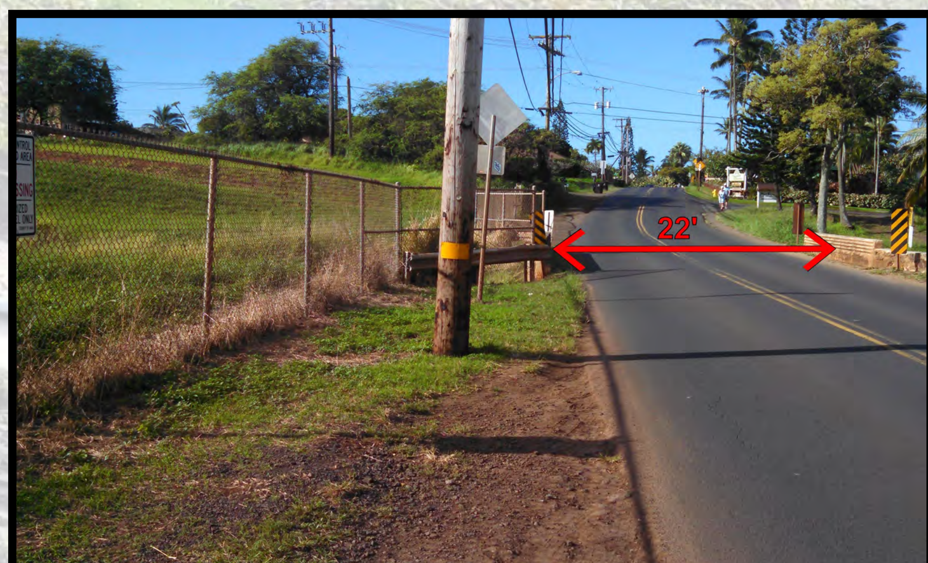
BEFORE: Narrow, 22-foot roadway crossing.
